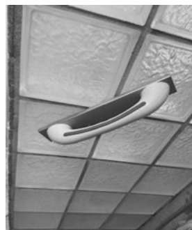
Glass block shower stall across grout lines
