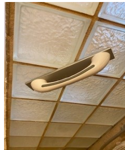
Glass block shower stall across grout lines
